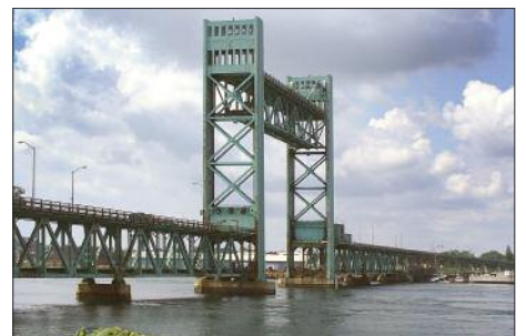
In 2009, the Durham based NECA member completed the project for the NH Dept. of Transportation and the Interstate Bridge Authority. It involved a complete upgrade of the Bridge's lift and control systems.
