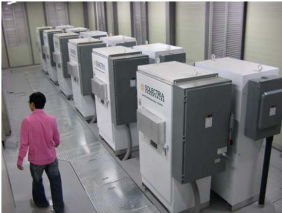
Solectria Renewables inverters up and running
